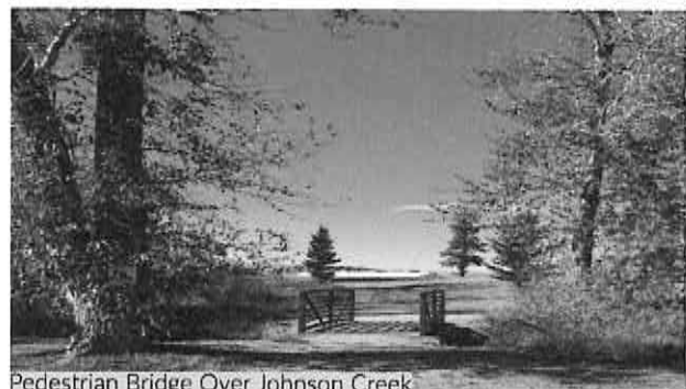
Pedestrian Bridge Over Johnson Creek
